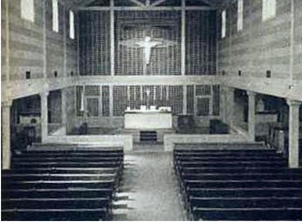
St. Francis of Assisi Church in Portland
